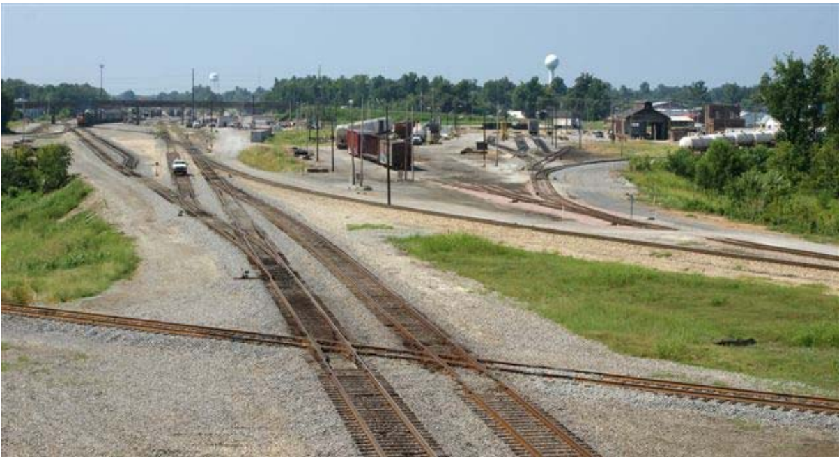
This is the new diamond (at Fulton, KY) recently reinstalled to support NS coal trains going to Nashville via Jackson TN. These are from fellow railfan and CN engineer Darren Doss.
